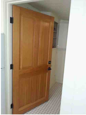
Upgraded Bathroom Door
